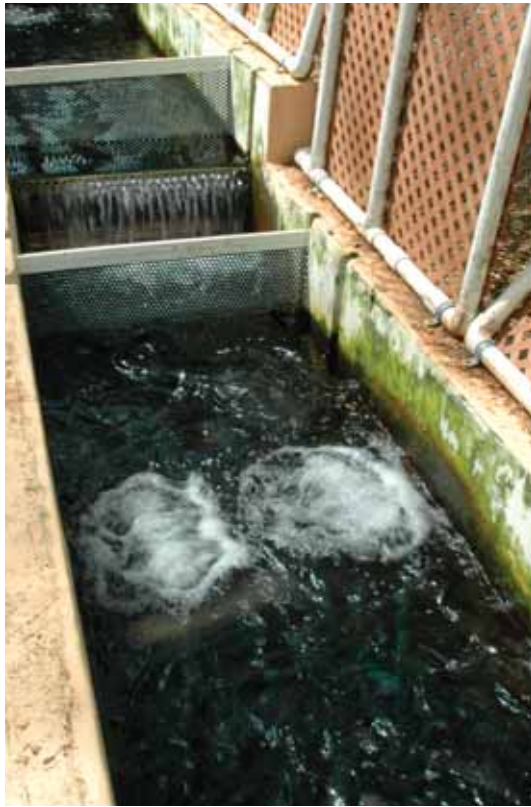
Stony Creek Trout Nursery's raceway is gunnite, the type of concrete used in swimming pools. Steps built into the raceway maximize water flow and aid in aeration.
